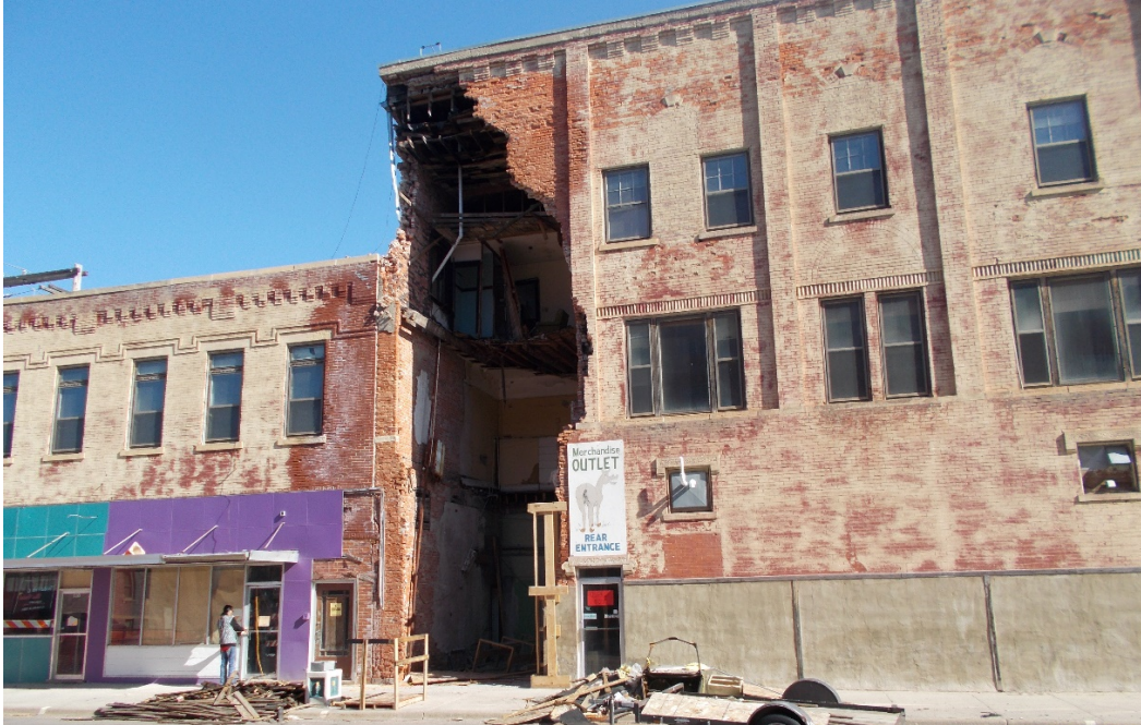
Figure 2. Photo showing condition of South wall on April 27, 2018
