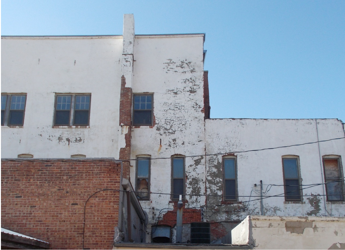
Figure 4. Photo of Northwest corner of East building.
