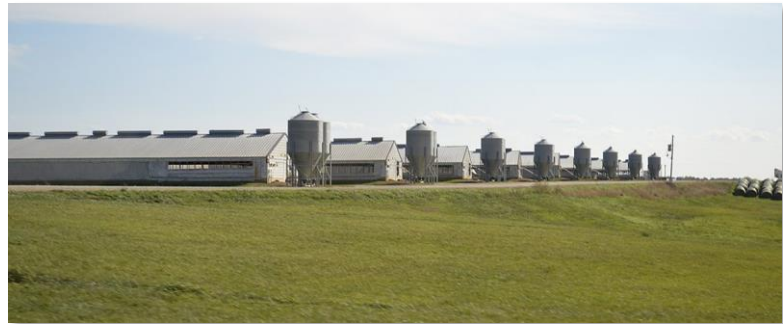
Hog Production Facility
