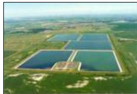
Mitchell Wastewater Treatment Facility
