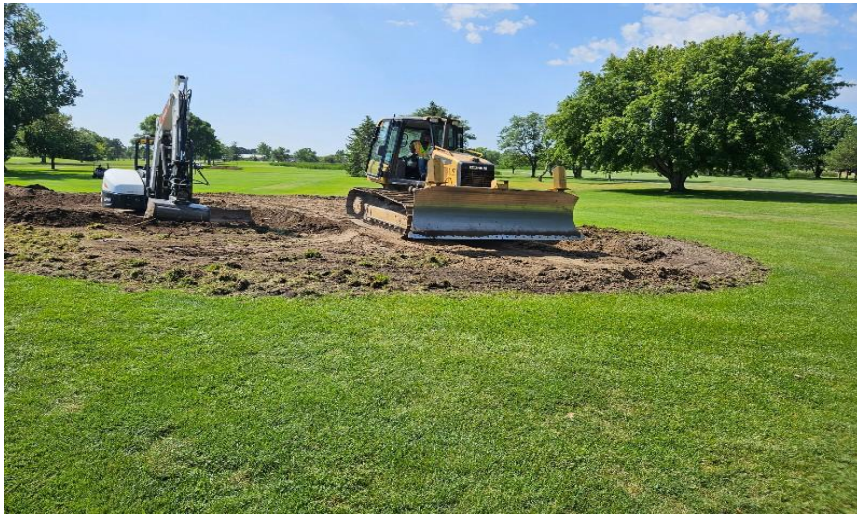
Starting to reshape #17 bunker.
