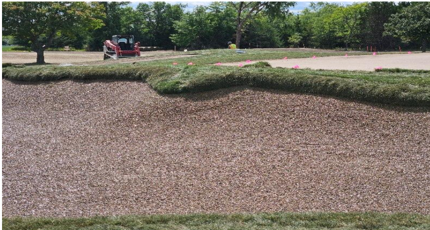
#14 bunker with bunker liner and sodded.
