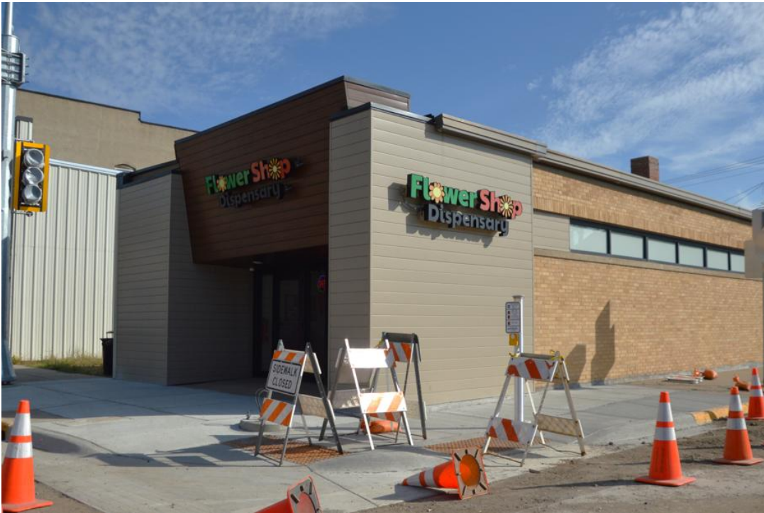
SD_Davison County_Mitchell Historic Commercial District (AD, BI, BD)_0002 View of 100 N. Main, camera looking northeast.
