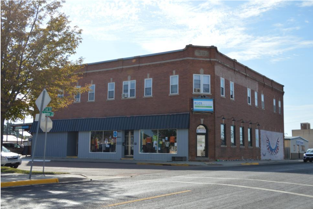
SD_Davison County_Mitchell Historic Commercial District (AD, BI, BD)_0007 View of 201 E. 2 nd Ave. at Lawler St. (Area of boundary decrease), camera looking southeast.
