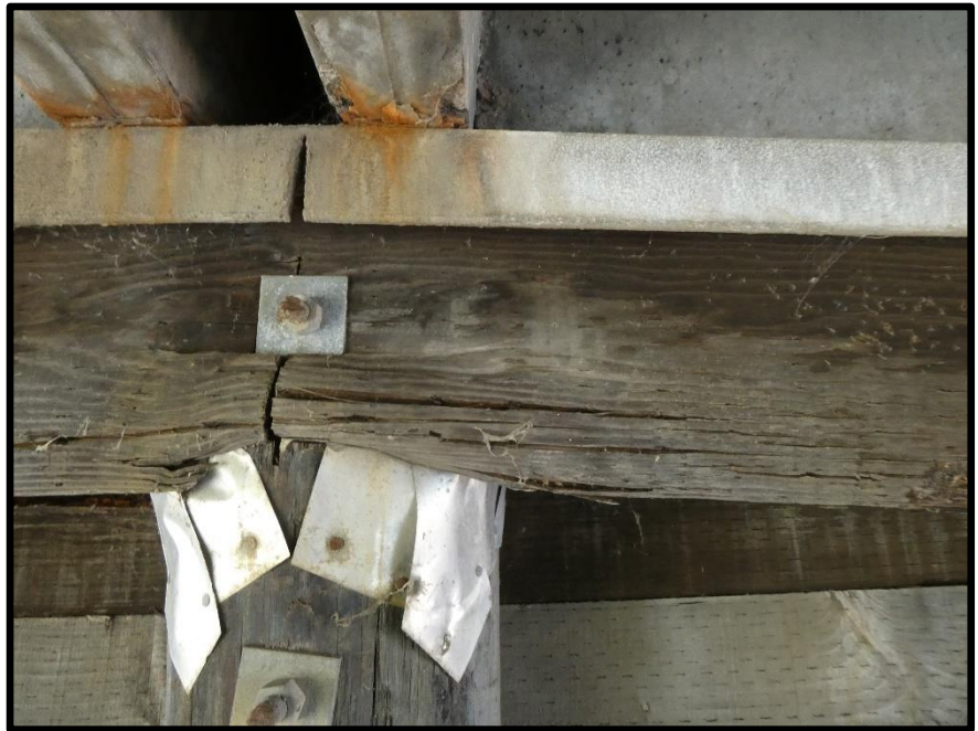
Crushing North Abutment Cap Over Pile 4
