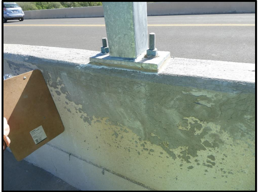
Typical Repair under Barrier Rail Posts
