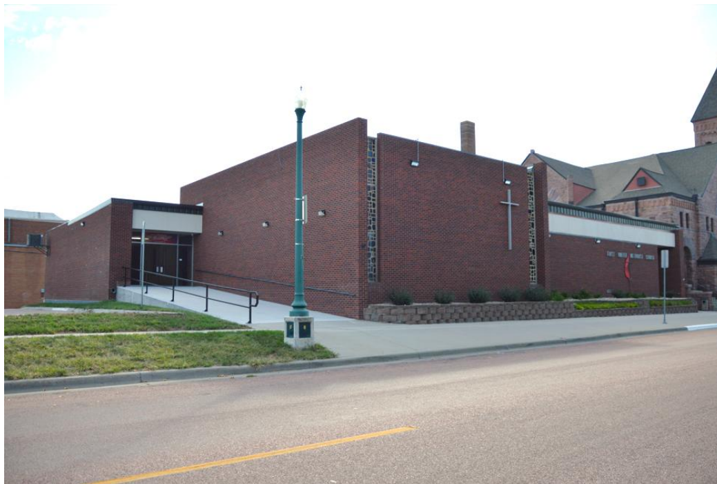
SD_Davison County_Mitchell Historic Commercial District (AD, BI, BD)_0012 View of First Methodist Church addition (Area of boundary increase), camera looking southeast. Date photographed: September 29, 2025.
