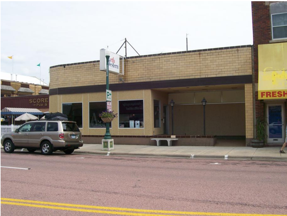
SD_Davison County_Mitchell Historic Commercial District (AD, BI, BD)_0007 “Before” view of 514 N. Main Street (edges of 512 and 522 N. Main – now demolished), camera looking east. Date photographed: September 3, 2008.
