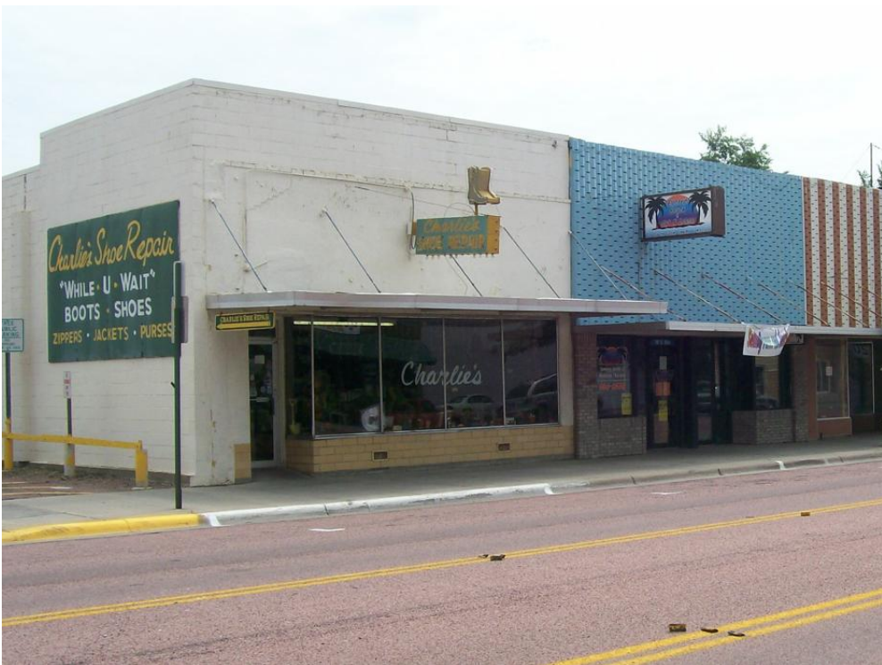
SD_Davison County_Mitchell Historic Commercial District (AD, BI, BD)_0005 "Before" view of 118 N. Main, camera looking southeast. Date photographed: September 3, 2008.
