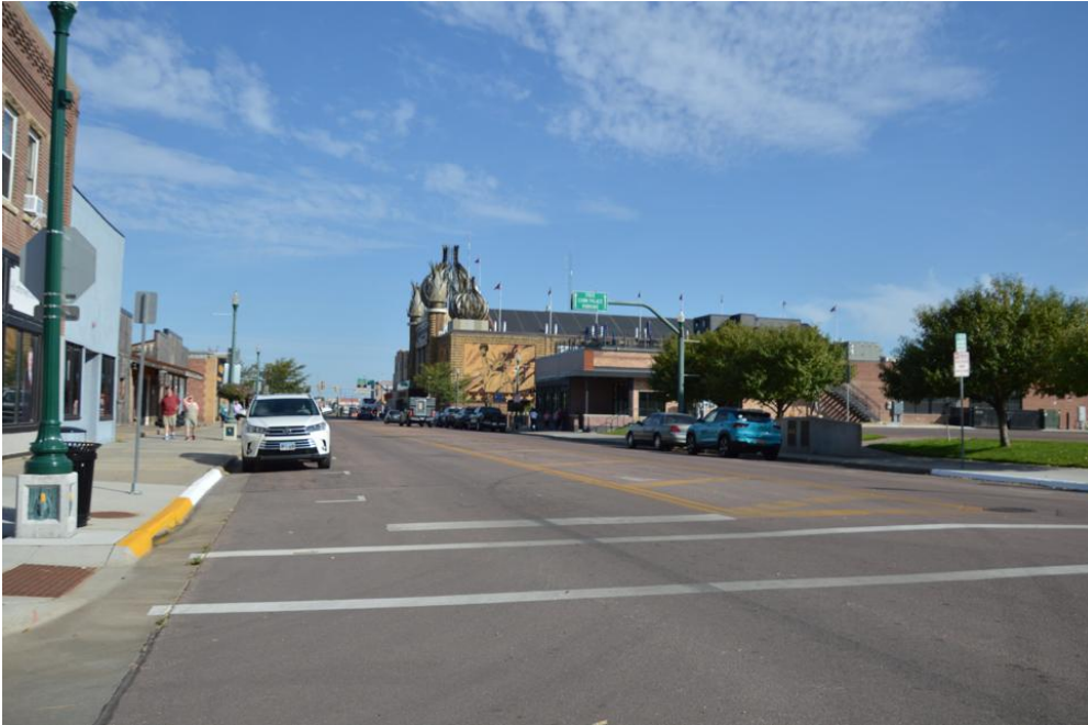
SD_Davison County_Mitchell Historic Commercial District (AD, BI, BD)_0006 View of 514 N. Main Street (512 and 522 N. Main – demolished) with Corn Palace in background, camera looking northeast. Date photographed: September 29, 2025.
