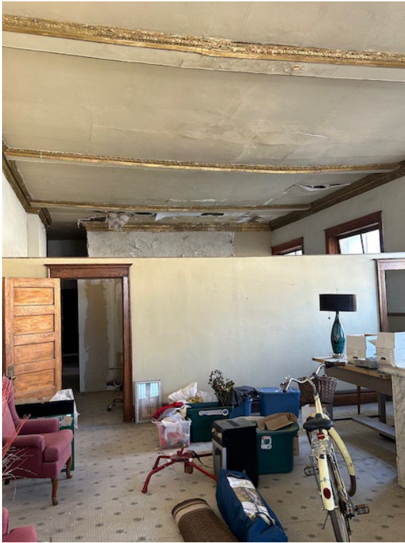
Inside front entrance facing West toward bank vault
