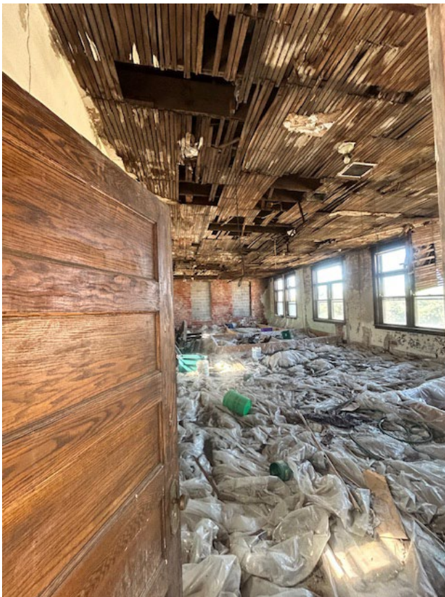
Top of 3 rd floor stair looking west
