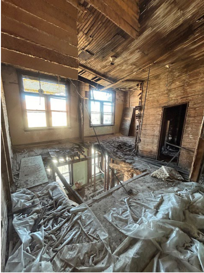
3rd floor looking north from the south hall
