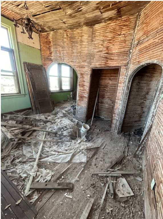
3rd floor looking toward the southeast
