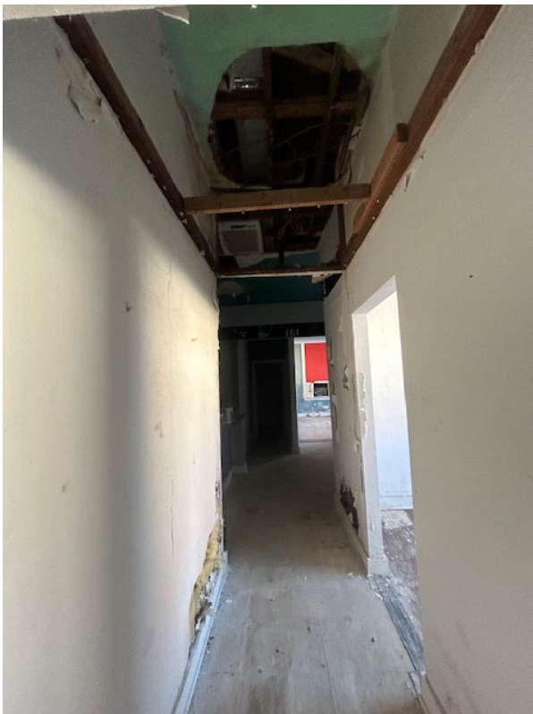
West end hall looking west toward alley
