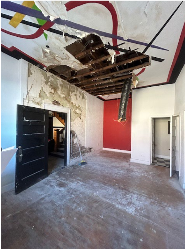
West end looking back to stair case and side entrance
