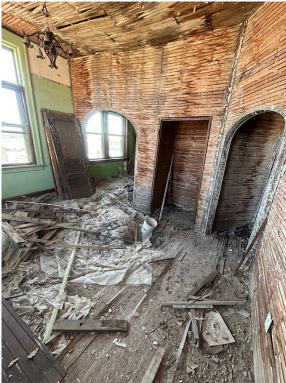
3rd floor looking toward the southeast
