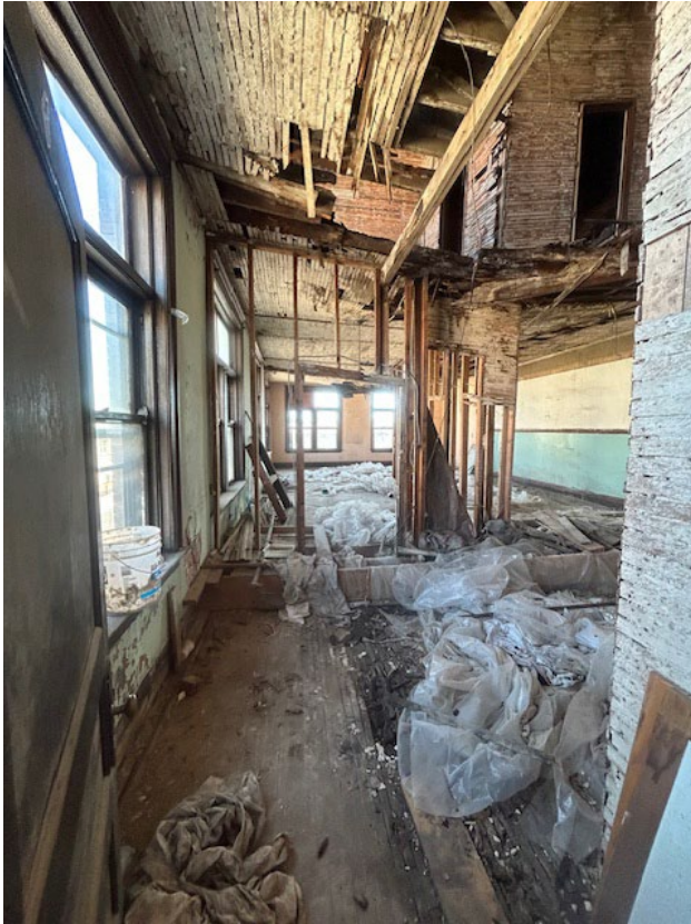
2 nd floor along south hall
