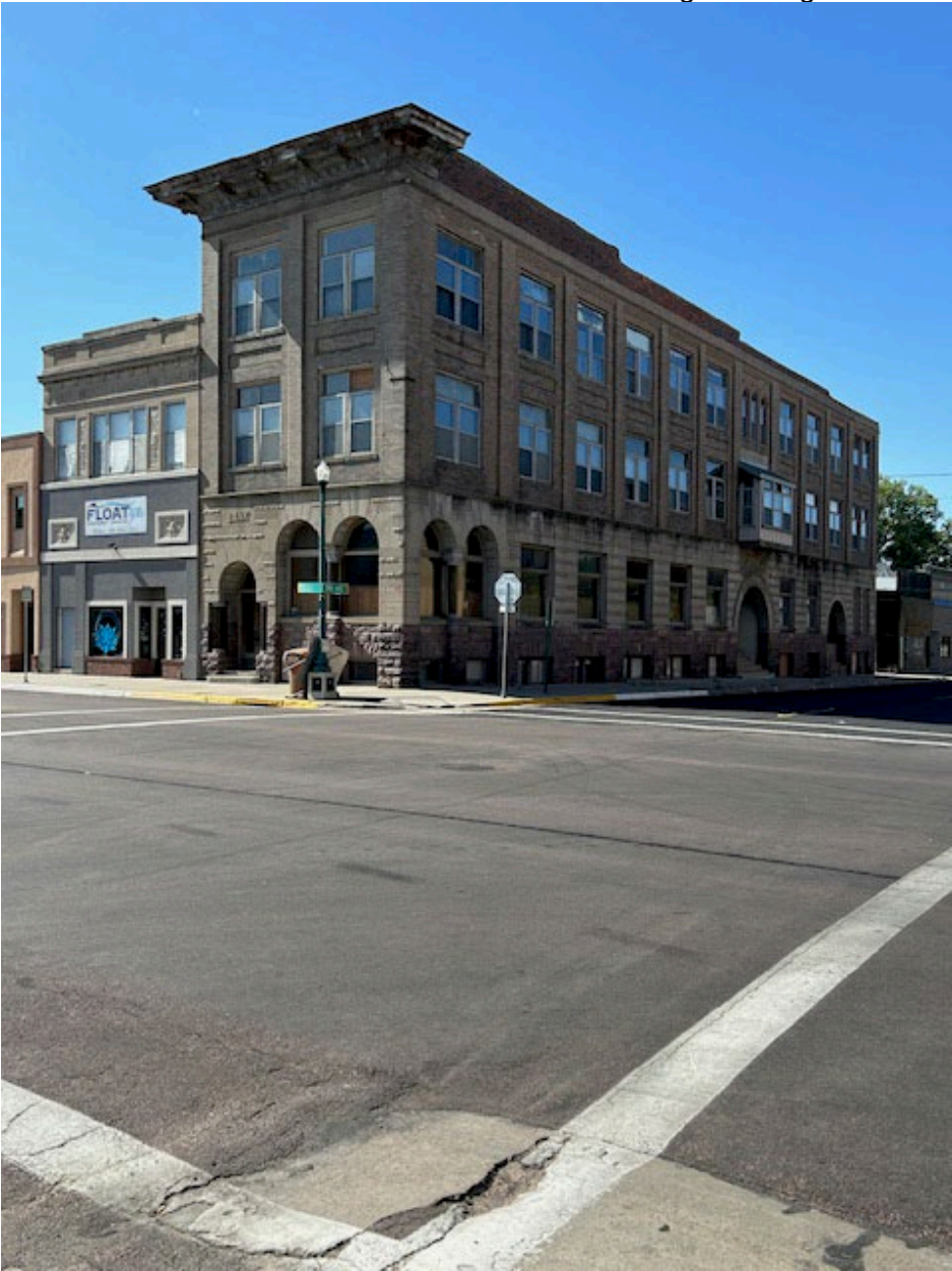
Norh East corner facing South West
