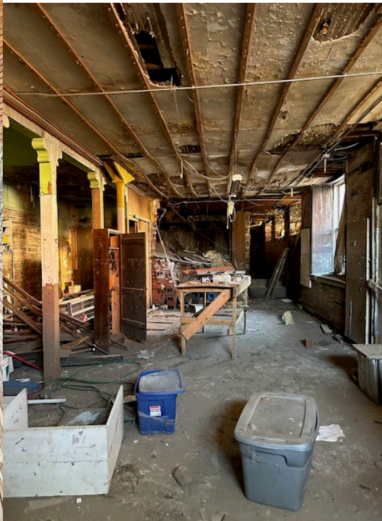
Basement end looking west
