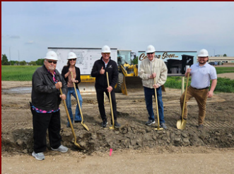
Groundbreaking at Chef Louie's
